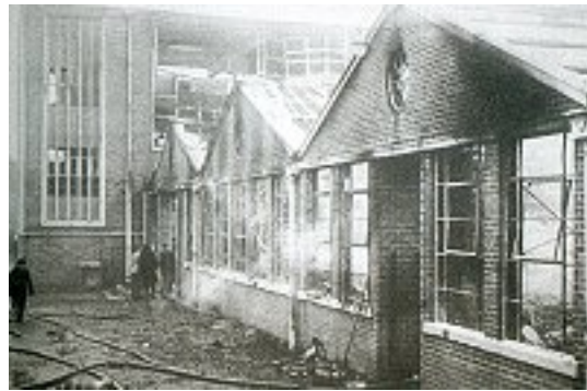
Factory fire: the remains of the Garrards factory after the 1958 blaze - still Swindon's biggest fire
