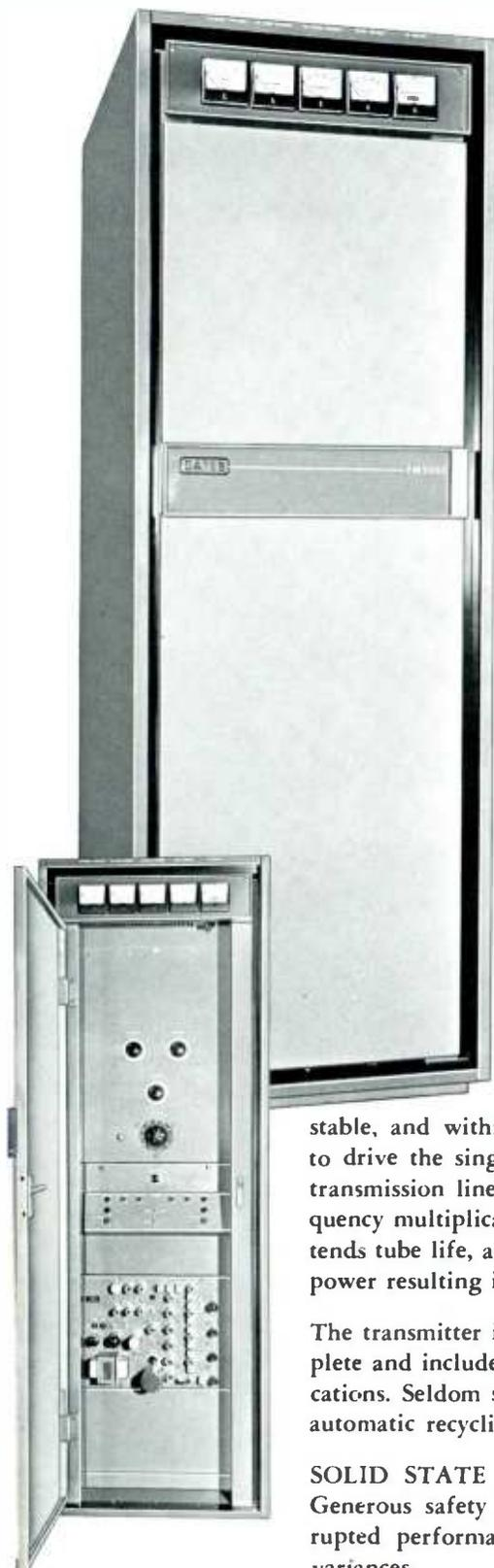
The more rigid requirements for stereo and multiplexing were seriously considered in the decisive action by Gates engineers to offer the industry an entirely new transmitter instead of a modification of an earlier model. Wider response, lower distortion, greatly improved channel separation for stereo, and low noise, combine to provide the richest quality sound in FM broadcasting.
