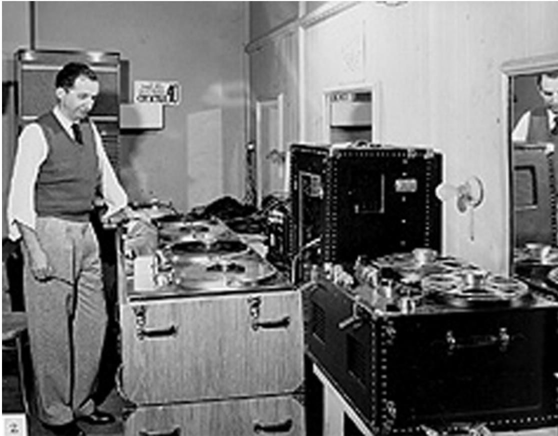
“Jack Mullin seen above in 1949 with the Ampex 200-A and the new Ampex 300 in portable cases, head blocks showing original tape backing facing in. This was later changed to the backing facing out, as it remained throughout the remainder of reel to reel production.” -MOMSR
